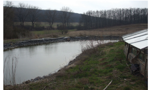
Figure 2.3: Water reservoir built to collect rainwater from the roof of a greenhouse, it reflects sunshine on the glasshouse and it is used for passively irrigating vegetable beds. Credit: Alfréd Szilágyi
